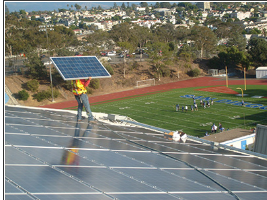
Photo: Courtesy of Main Street Power Company Inc. A solar panel is installed on the roof of a San Diego High School building in San Diego, Calif., one of 100 rooftops on which solar energy systems were installed as part of the San Diego Unified School District project.
